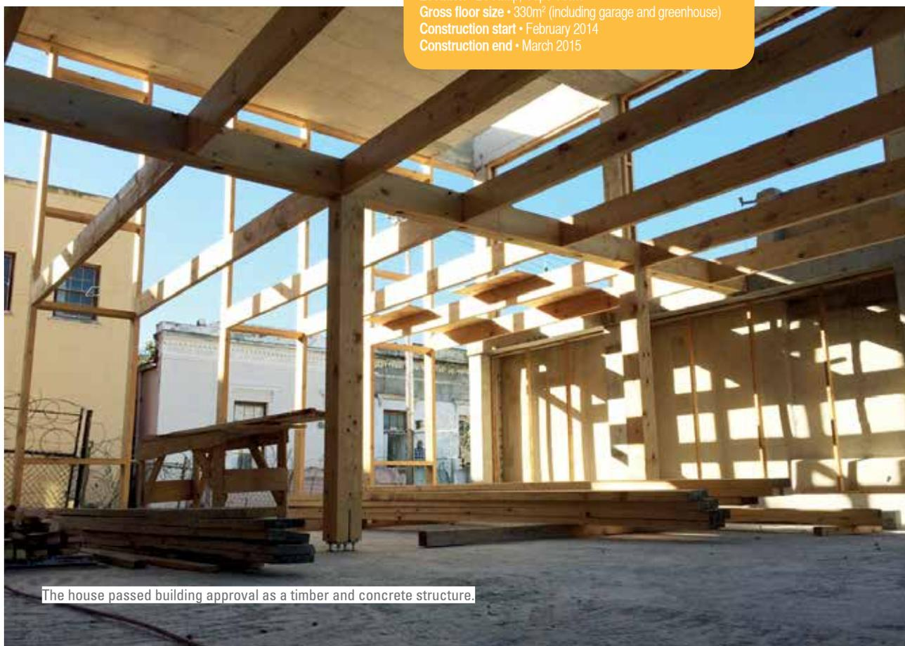
The house passed building approval as a timber and concrete structure.
